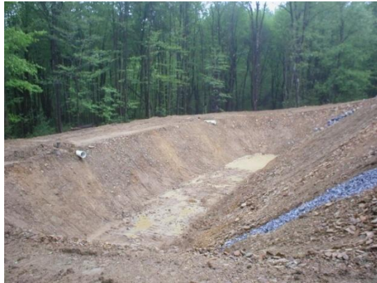
Excavated polishing pond
