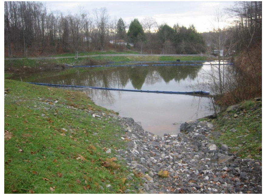
Pond and new pipe after reclamation
